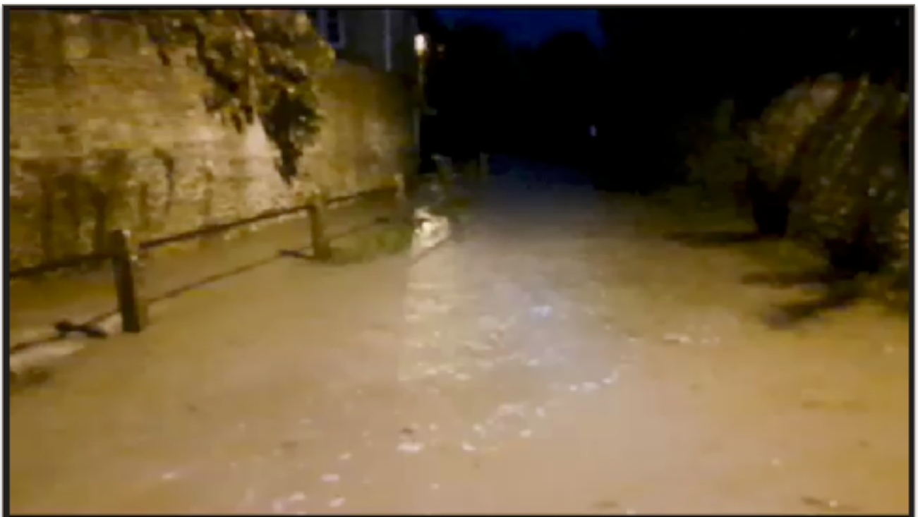
Flooding on Ringwell Lane January 2024
