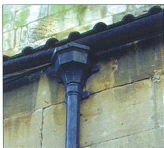
A cast iron rain water pipe
